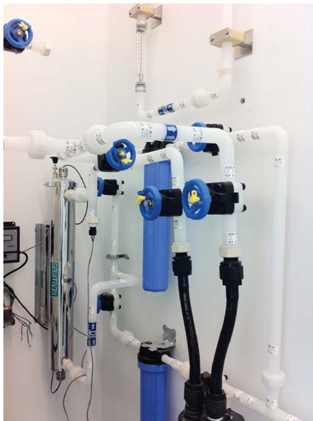
Asahi/America's Purad™ PVDF piping system with beadless welds for a pharmaceutical highly purified water system.
