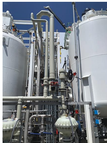
IMAGE 2: Glass-filled polyamide pneumatic actuators automating Type-21 ball valves in a lithium nickel slurry application.
