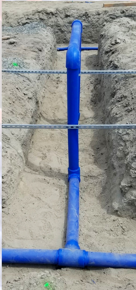
Air-Pro® in a buried application.
