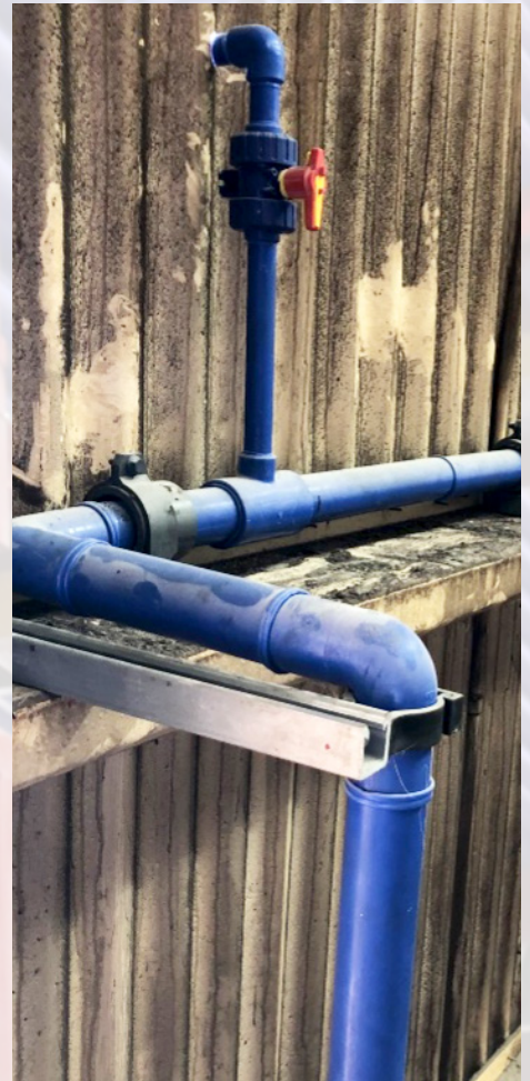
Air-Pro® at a fertilizer manufacturing facility covered in chemical dust.
