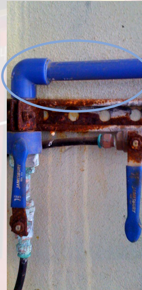
Air-Pro® at a bleach plant without corrosion.
