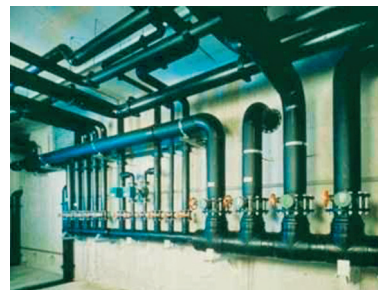
Figure 1. PE pipe installation
